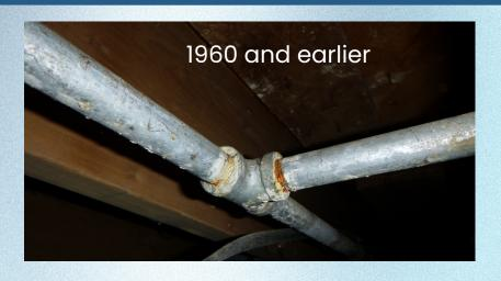
Galvanized Steel Water Supply Lines (dull gray/silver): Commonly installed in homes built before 1960. Based on its age alone, be aware that this material has exceeded its intended design life and will need to be replaced soon.
