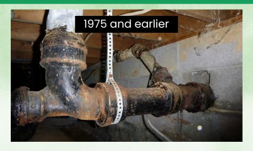
Cast Iron Drain/Waste Lines (black or rusted in appearance):
