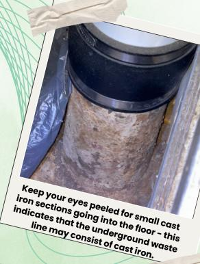
Before buying a house built prior to 1975, ALWAYS get the waste line scoped with a camera.
